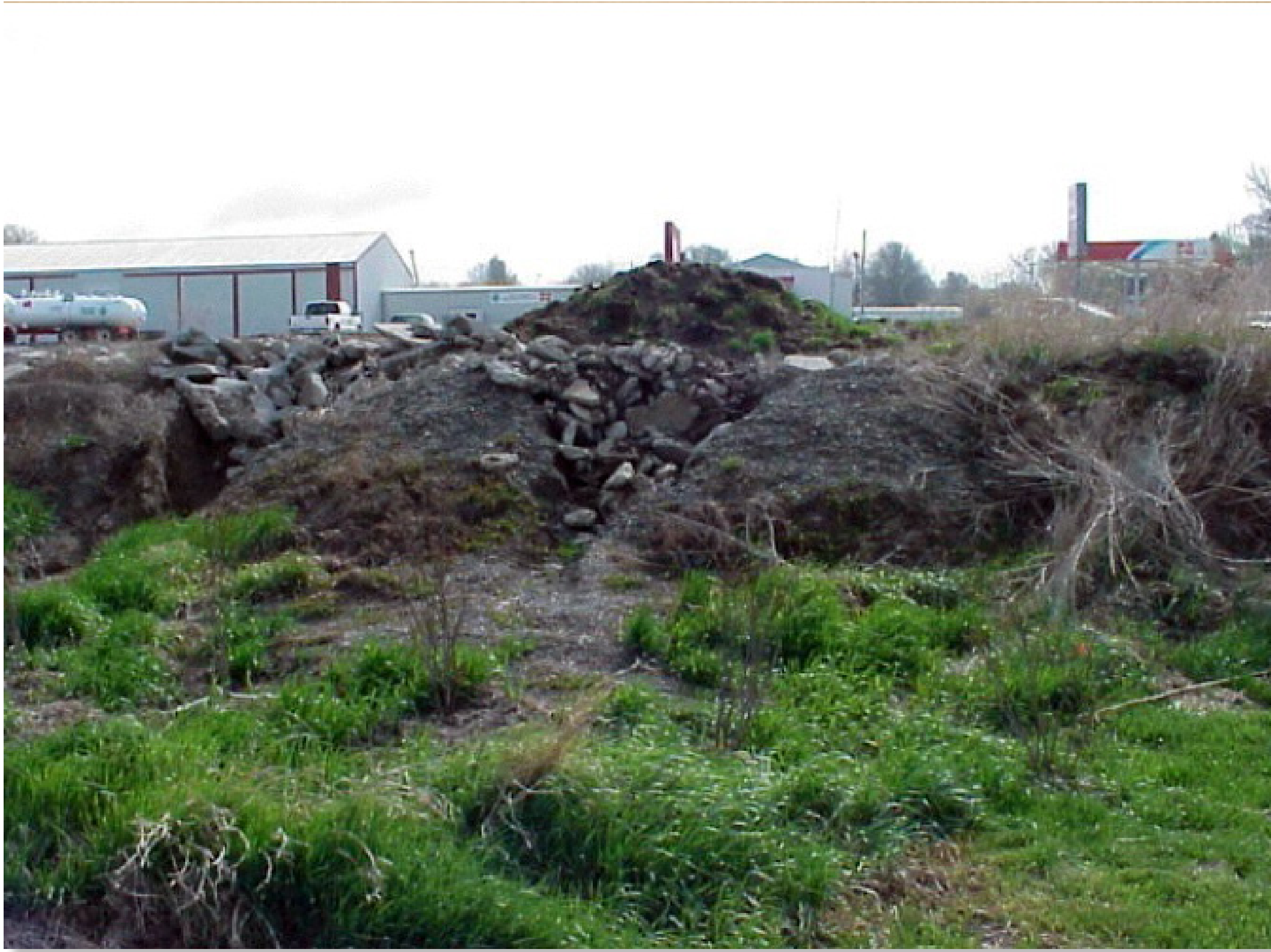
The north entrance corridor to Villisca on US 71 was filled with debris and suffering extreme erosion
